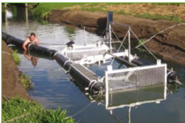
Installation of the Bandalong Floating Litter Trap.
