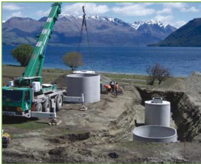
Installation of the precast tanks
