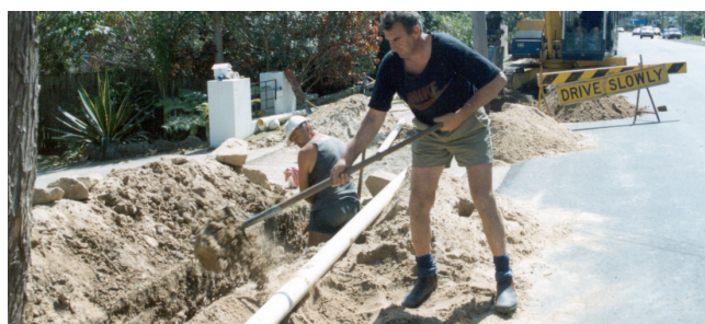
INSTALLATION: Shallow trenches ensure low installation costs.
