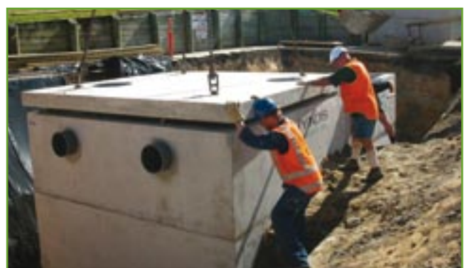
Hynds sand filter being installed.
