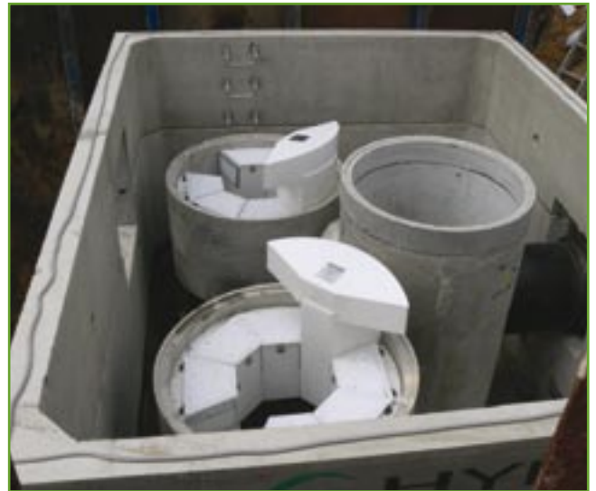
Installation of the Hynds UpFlo Vault.
